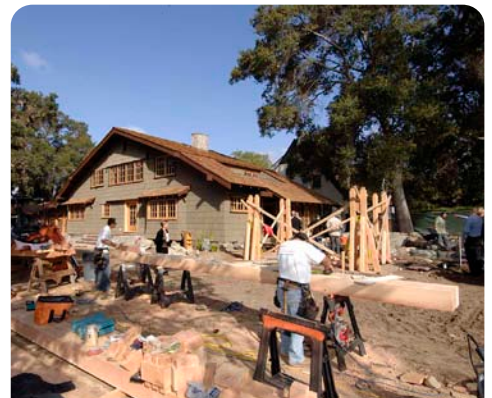
All cardboard, metal and concrete construction debris is recycled.
